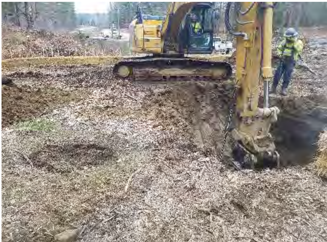
Fig 2: Beginning to excavate foundation for Str. 93. Viewing southeast. (04-09-20).
