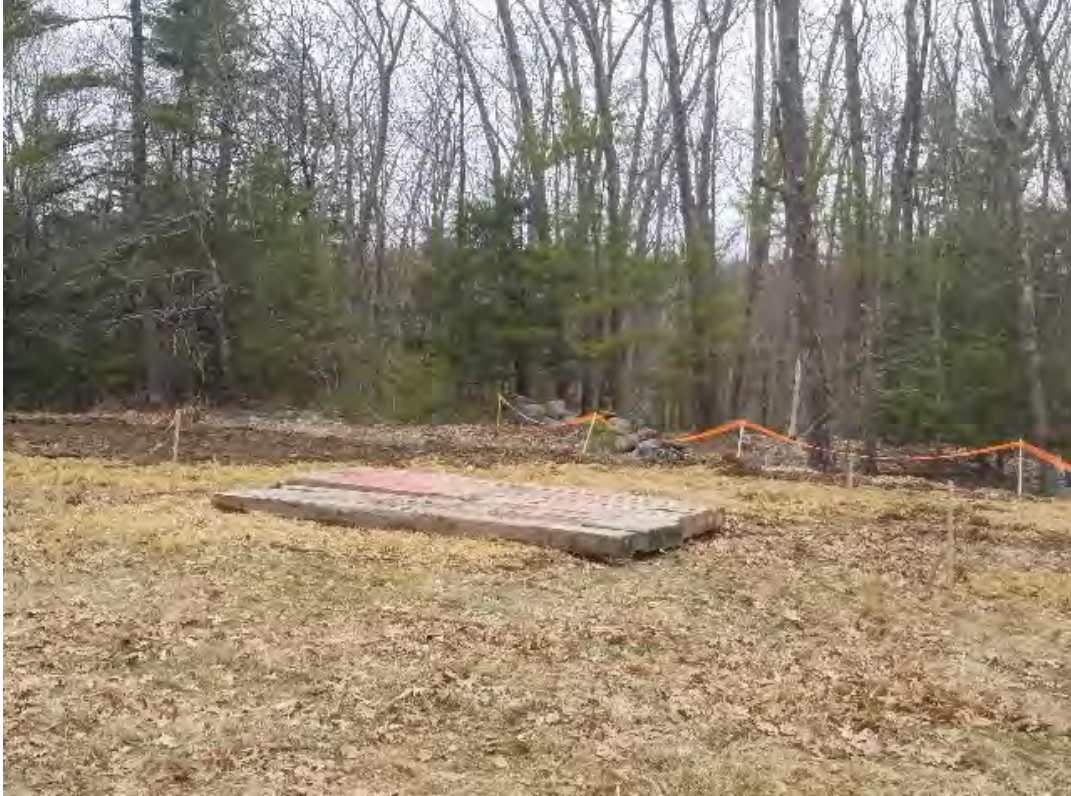
Fig 3: Foundation can set at Str. 92. Viewing north. (04-09-20).
