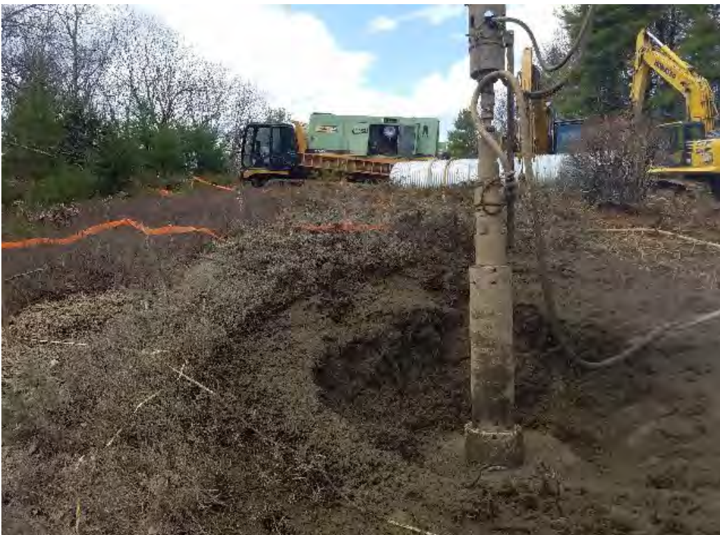
Fig 8: Drilling ledge for Str. 80 foundation. Viewing west. (04-15-20).
