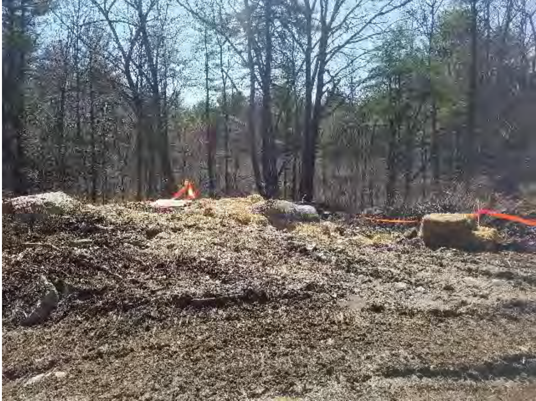
Fig 5: Foundation can set for Str. 79. Viewing southeast. (04-14-20).
