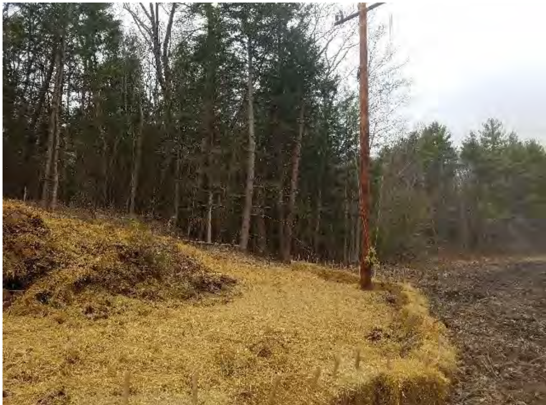
Fig 4: Distribution pole 3162-51 set. Viewing west. (04-09-20).
