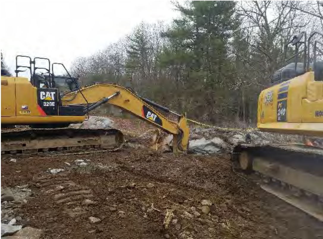
Fig 1: Hammering ledge at Str. 79. Viewing east. (04-09-20).
