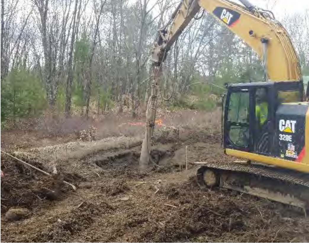
Fig 7: Drilling ledge at Str. 80. Viewing south. (04-15-20).
